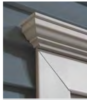
Crown molding is a classic accent to top off door or window trim.
